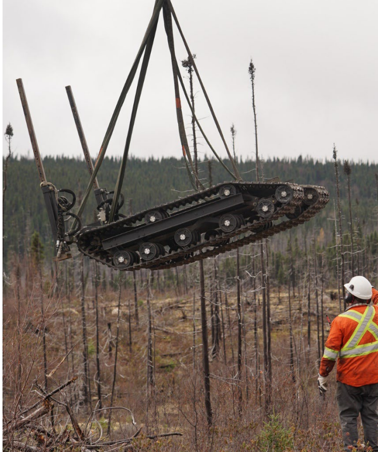
Figure 1: Drill mobilization at Red Mountain
